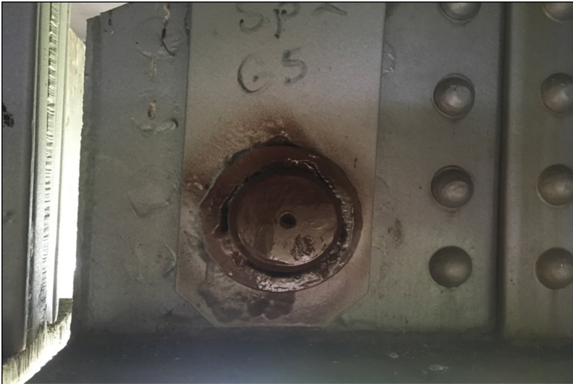
Span 2, Girder 5, Bottom Pin: Keeper missing washer is welded.
