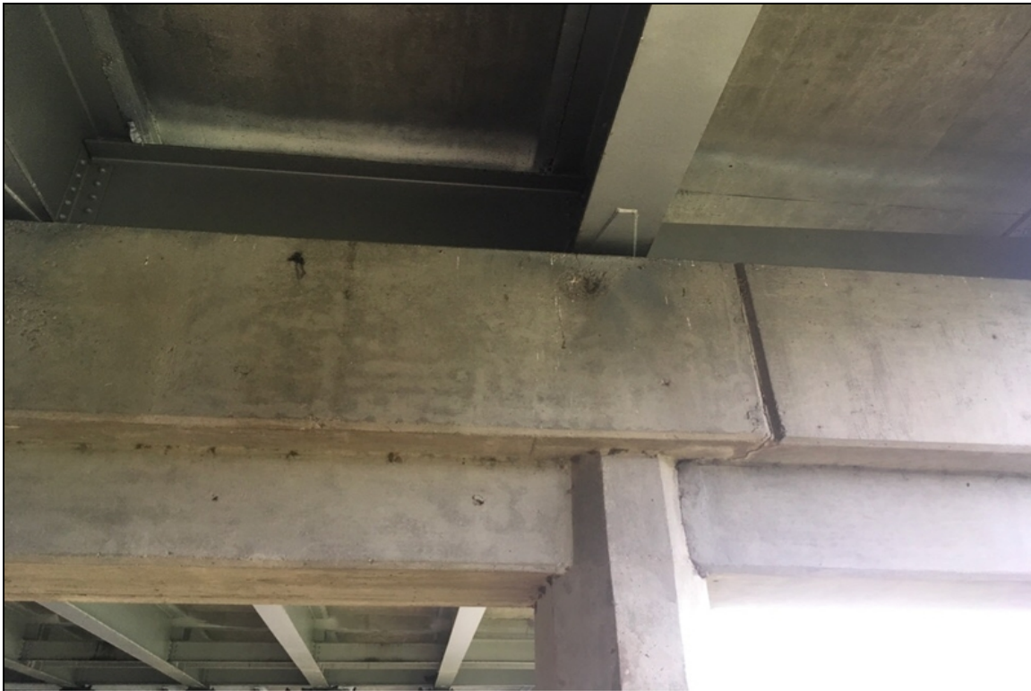
Bent 2, Girder 7, Cap: Minor spalling with exposed reinforcing steel.
