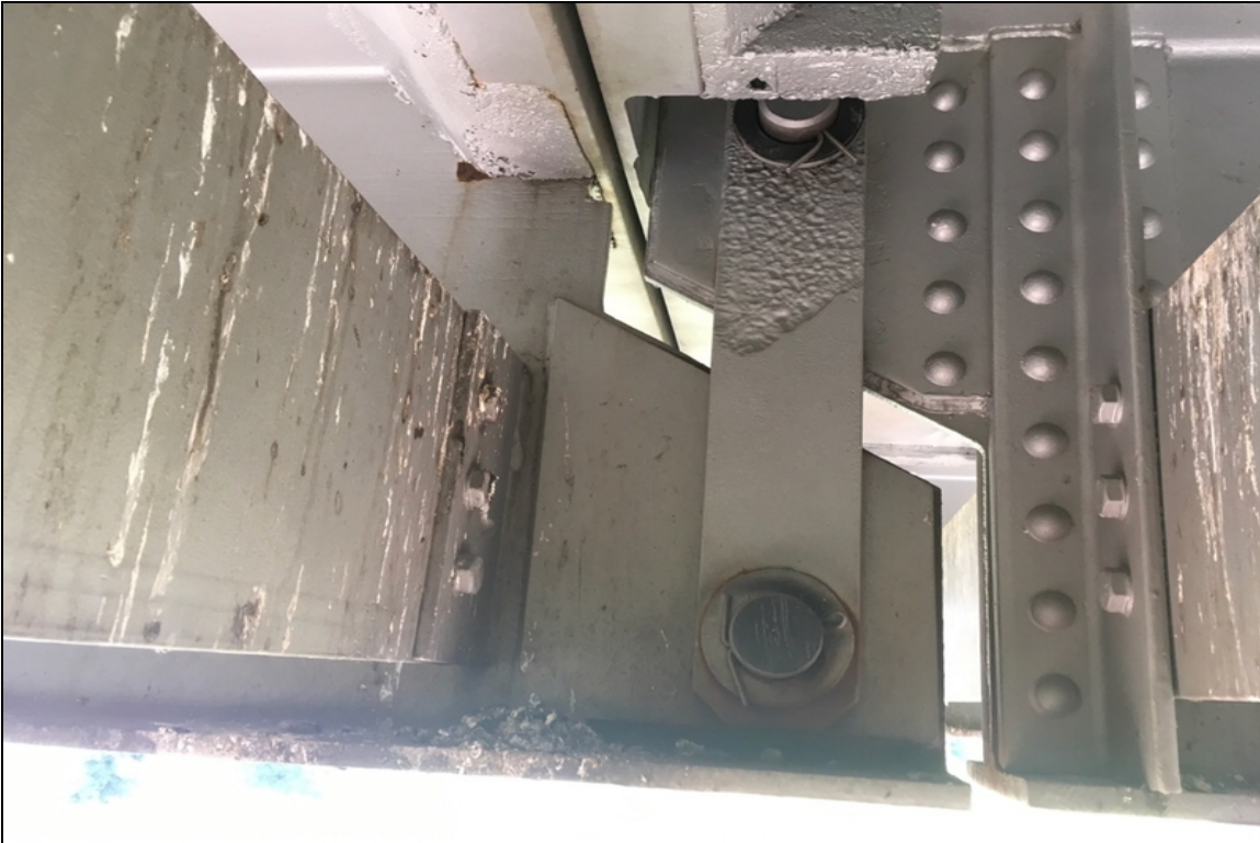
Span 18, Girder 7, Pin & Hanger: Floating.
