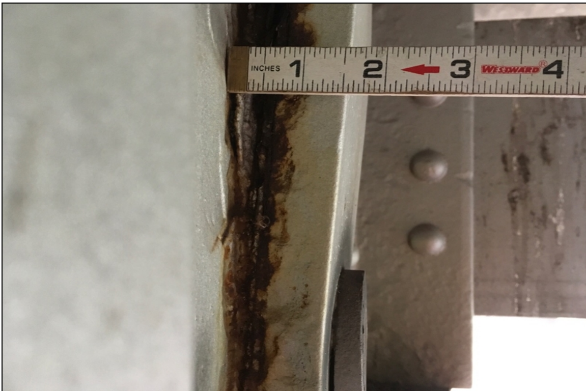
Span 3, Girder 6, Left, Hanger Bar: Out of plane bending.
