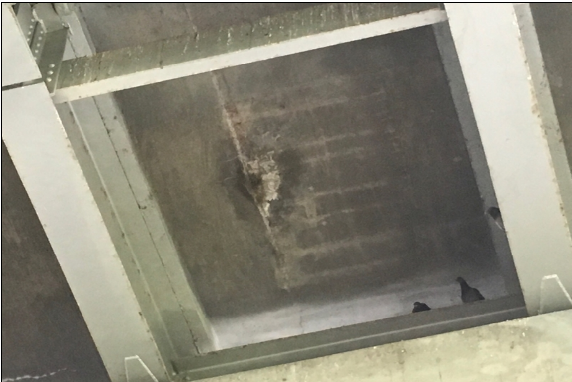
Span 3, Bay 4: Spalling.
