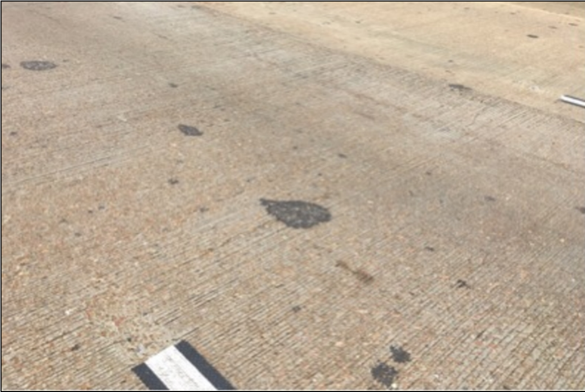
Span 8: Sealable deck cracking.
