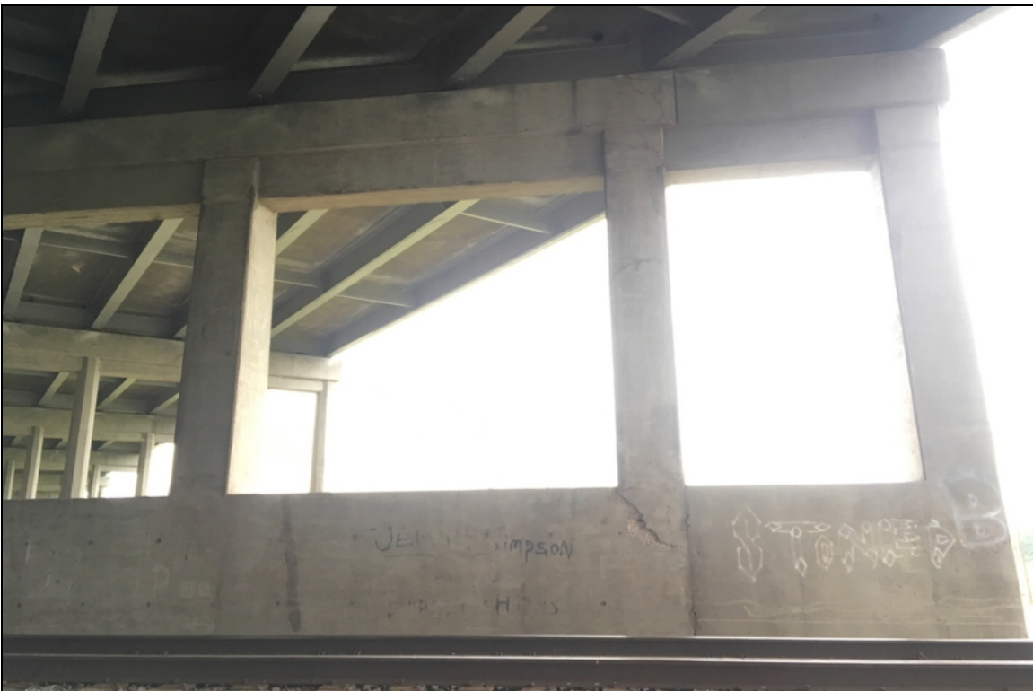
Bent 12, Column 5: Spalling.
