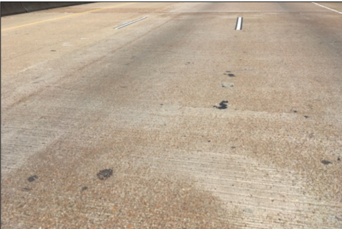
Span 17: Sealable transverse cracks.
