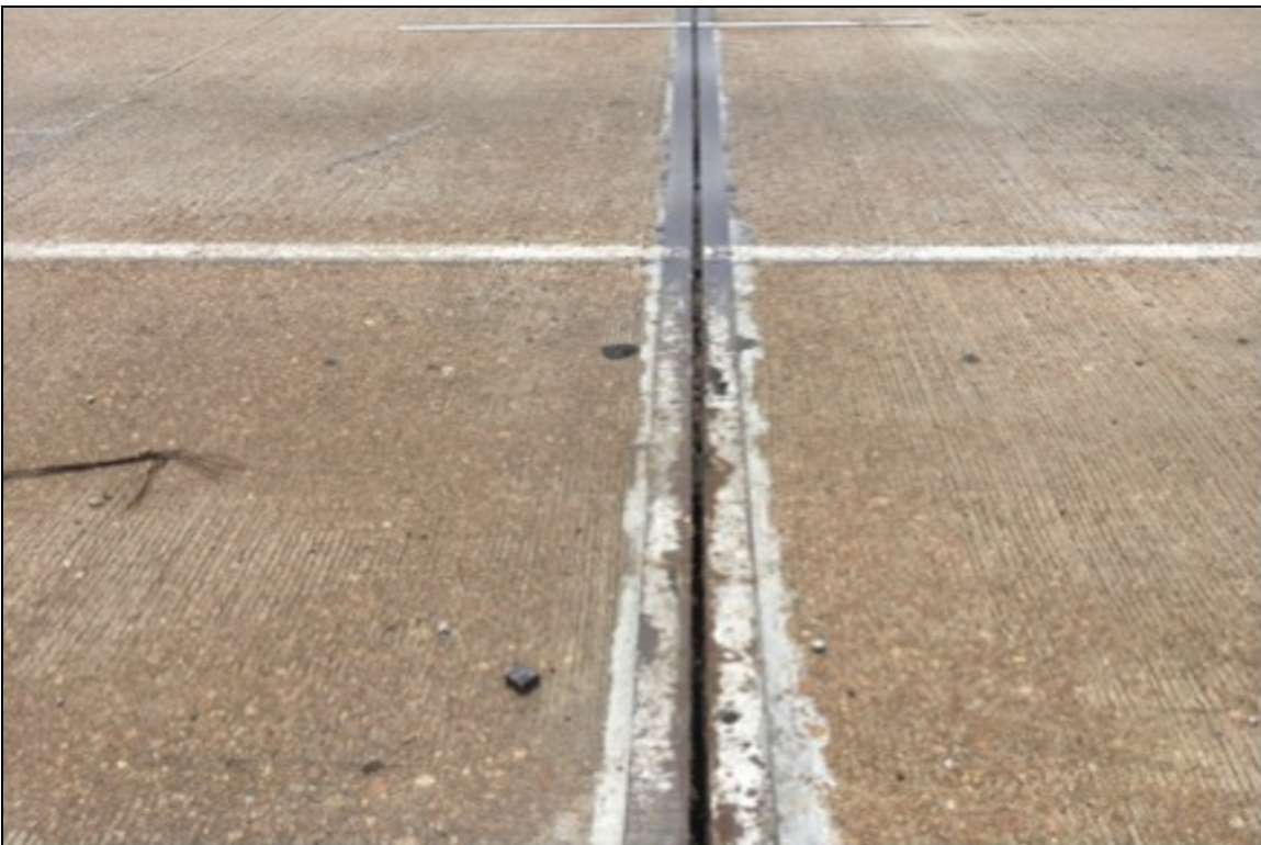
Span 14, Joint: Missing.
