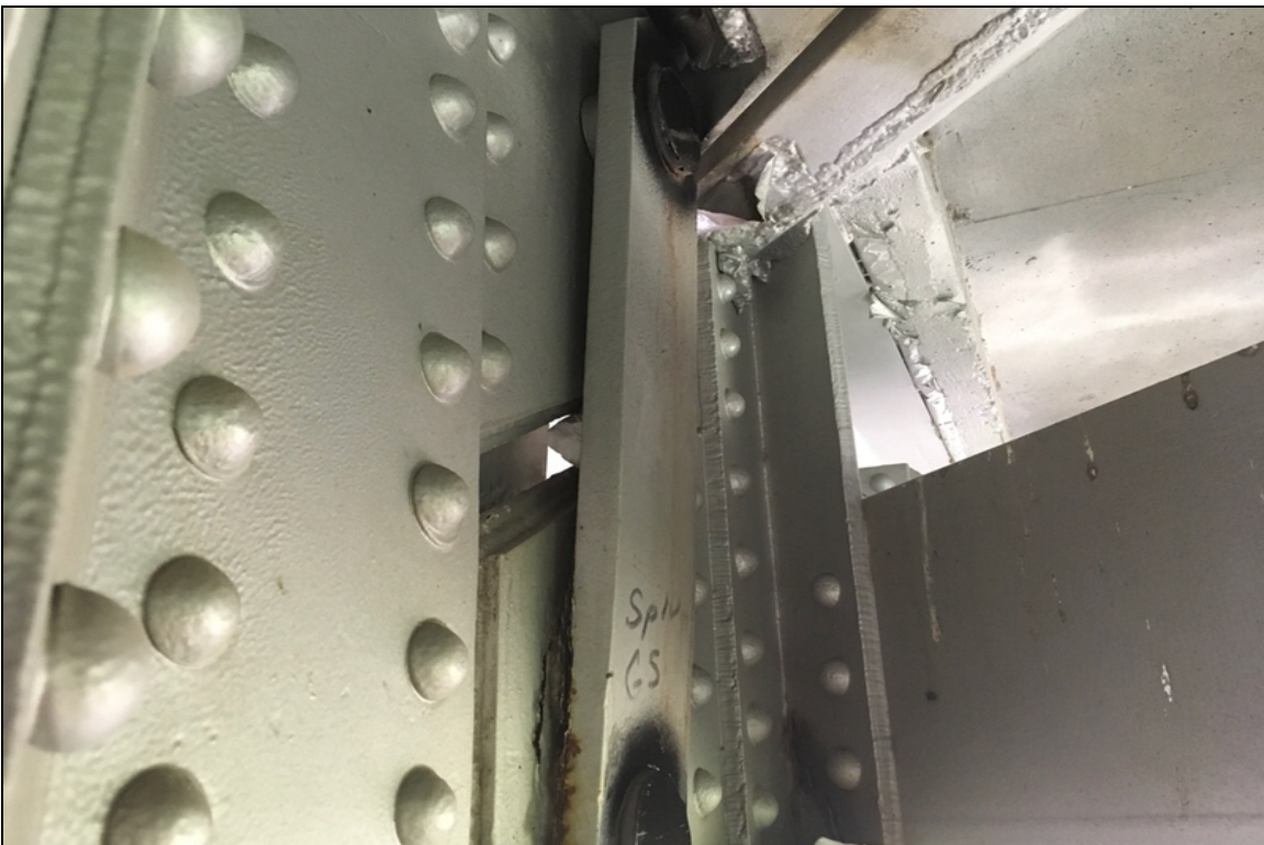
Span 10, Girder 5, Hanger Bar: Bulging.
