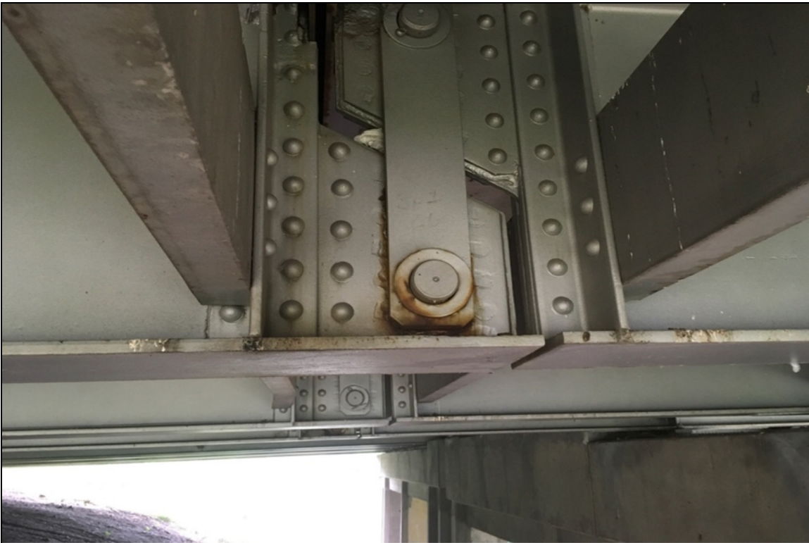
Span 1, Girder 6, Bottom Pin: Keeper missing washer is loose.
