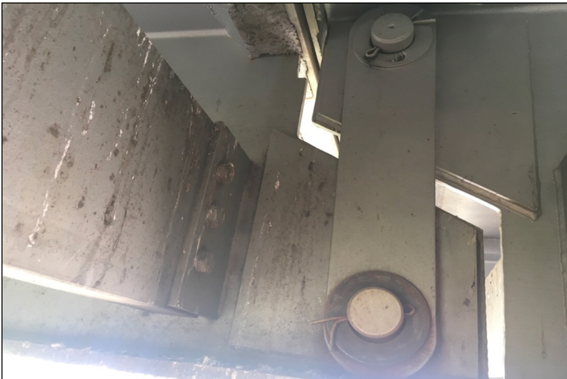
Span 20, Girder 4, Pin & Hanger: Floating.
