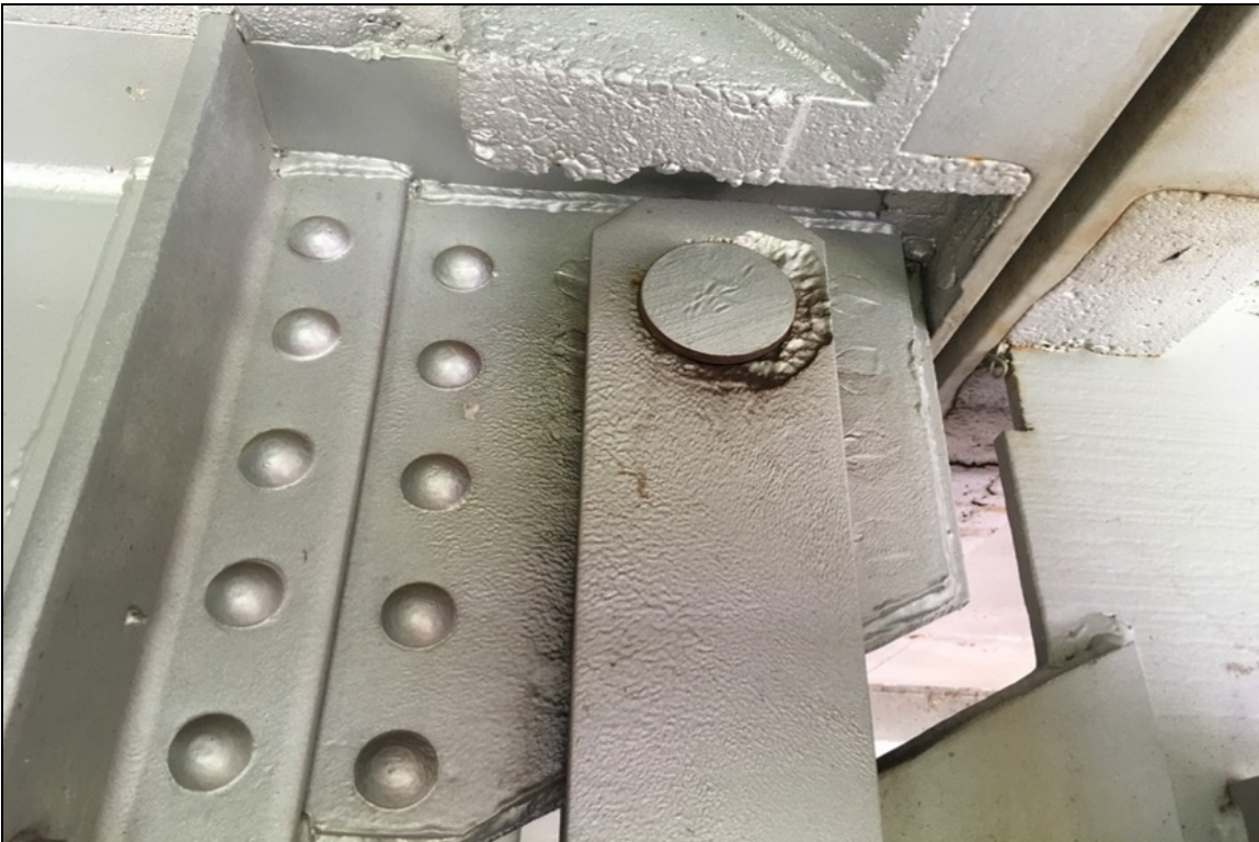
Span 18, Girder 9, Pin & Hanger: Floating.
