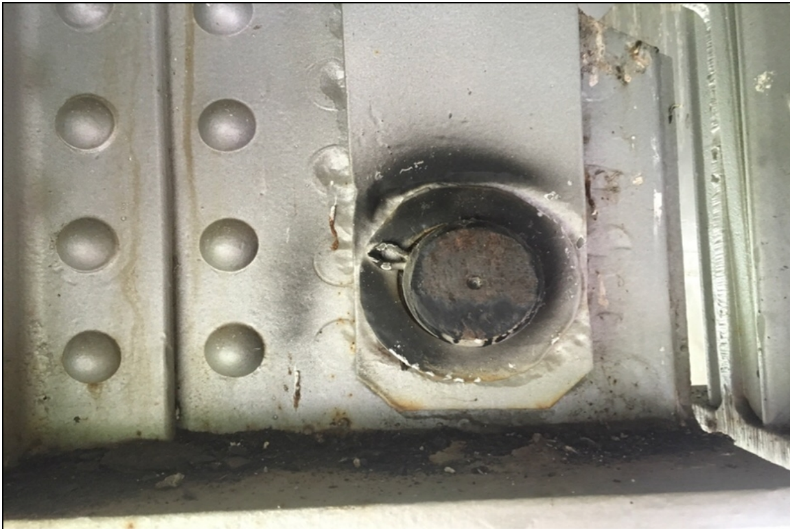
Span 3, Girder 4, Keeper: Sheared.
