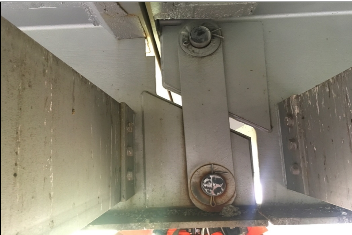
Span 21, Girder 6, Pin & Hanger: Floating.
