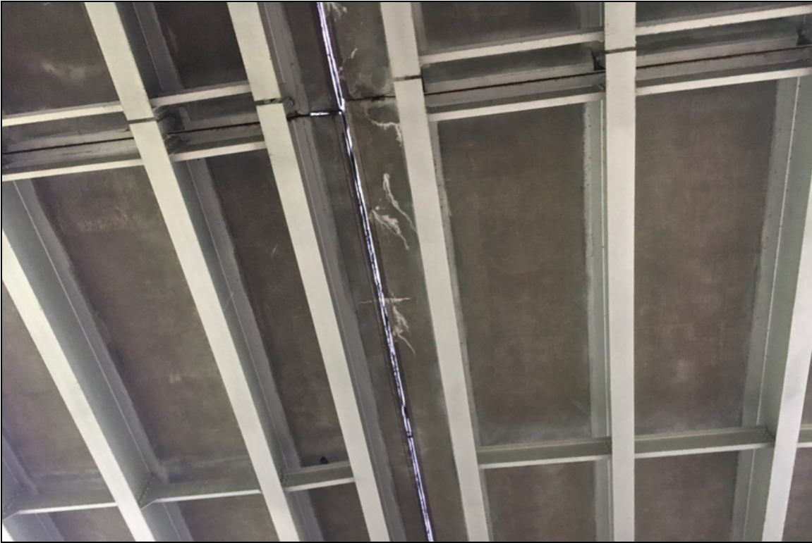
Span 17, Overhang, Left: Cracking with efflorescence.
