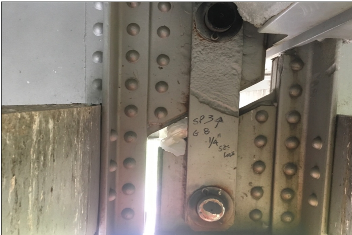
Span 3, Girder 8: Old section loss up to 1/4".
