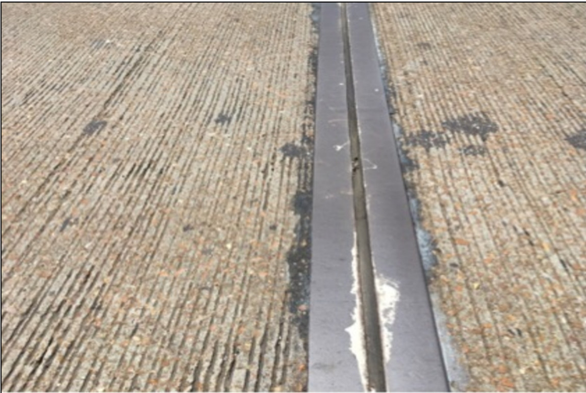
Span 4, Joint: 2' leakage.
