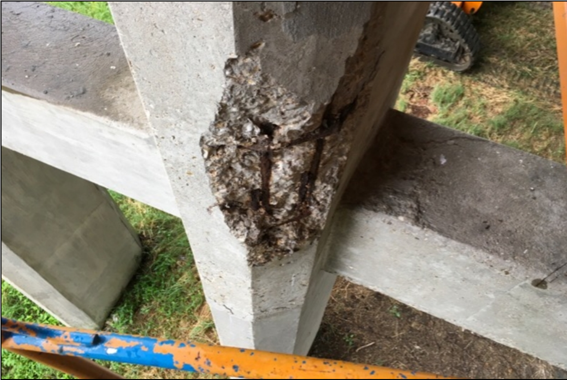
Bent 14, Column 5: Spalling with exposed reinforcing steel with section loss.
