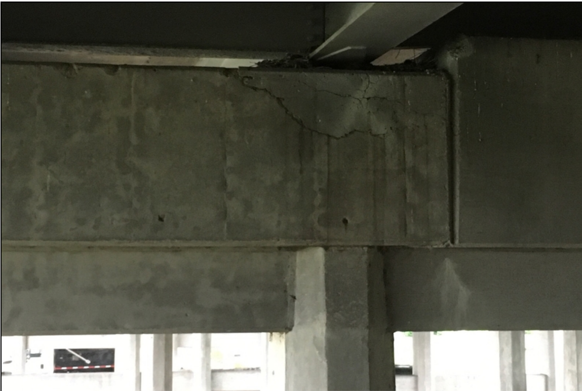
Bent 21, Girder 4: Delaminated repair.
