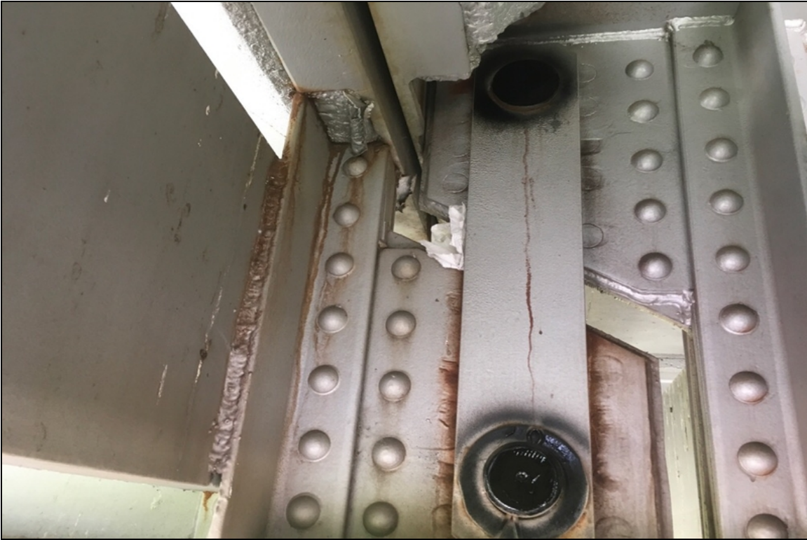
Span 8, Girder 8, Pin & Hanger: Floating.
