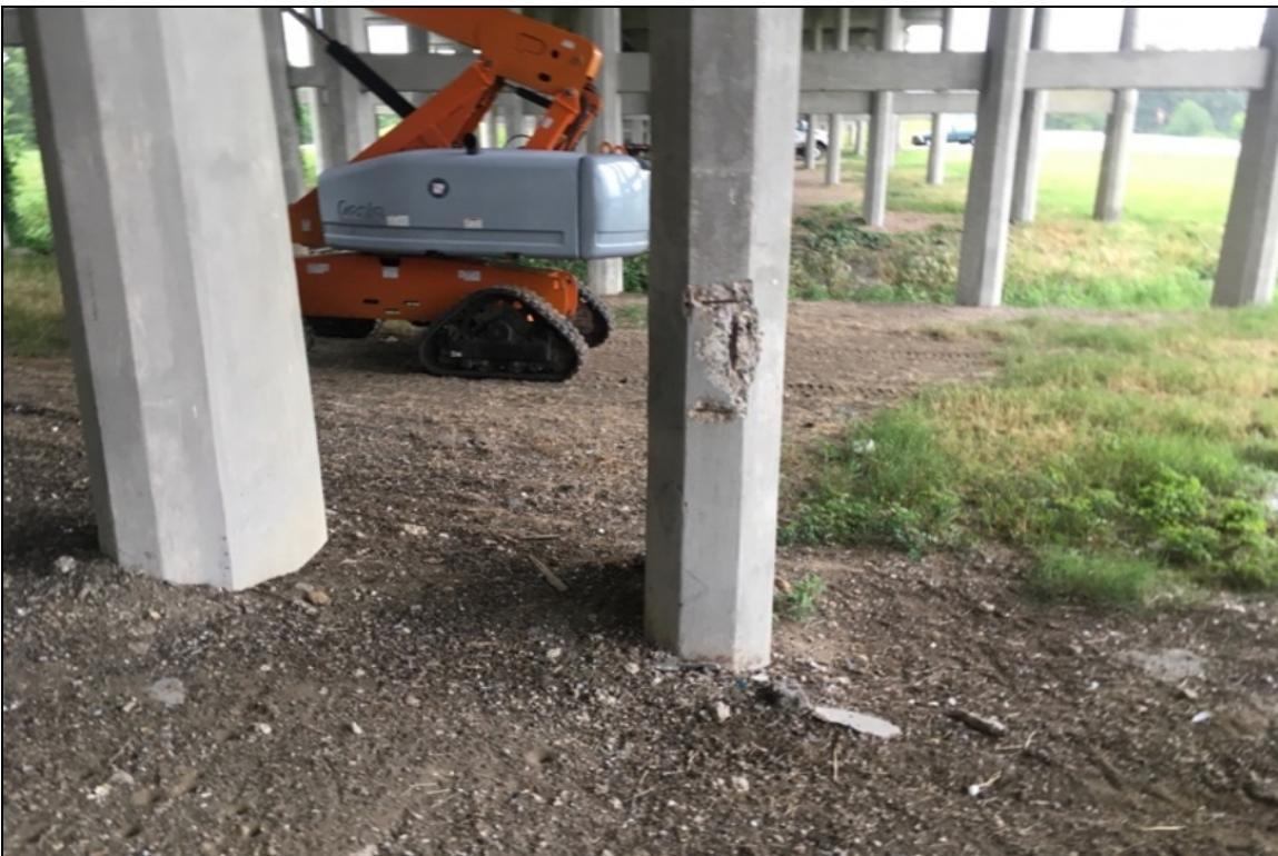
Bent 13, Column 3: Spalling with exposed reinforcing steel.
