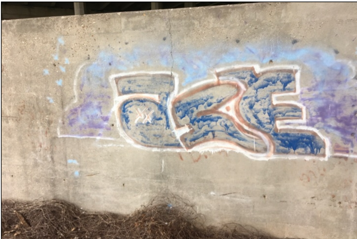
Bent 11, Pier Wall: Vertical cracking.
