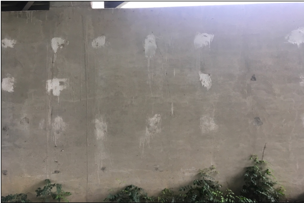
Pier Walls: Typical cracking.
