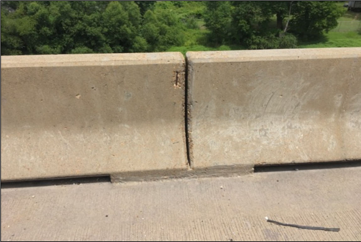
Bridge Rail: Typical exposed reinforcing steel.
