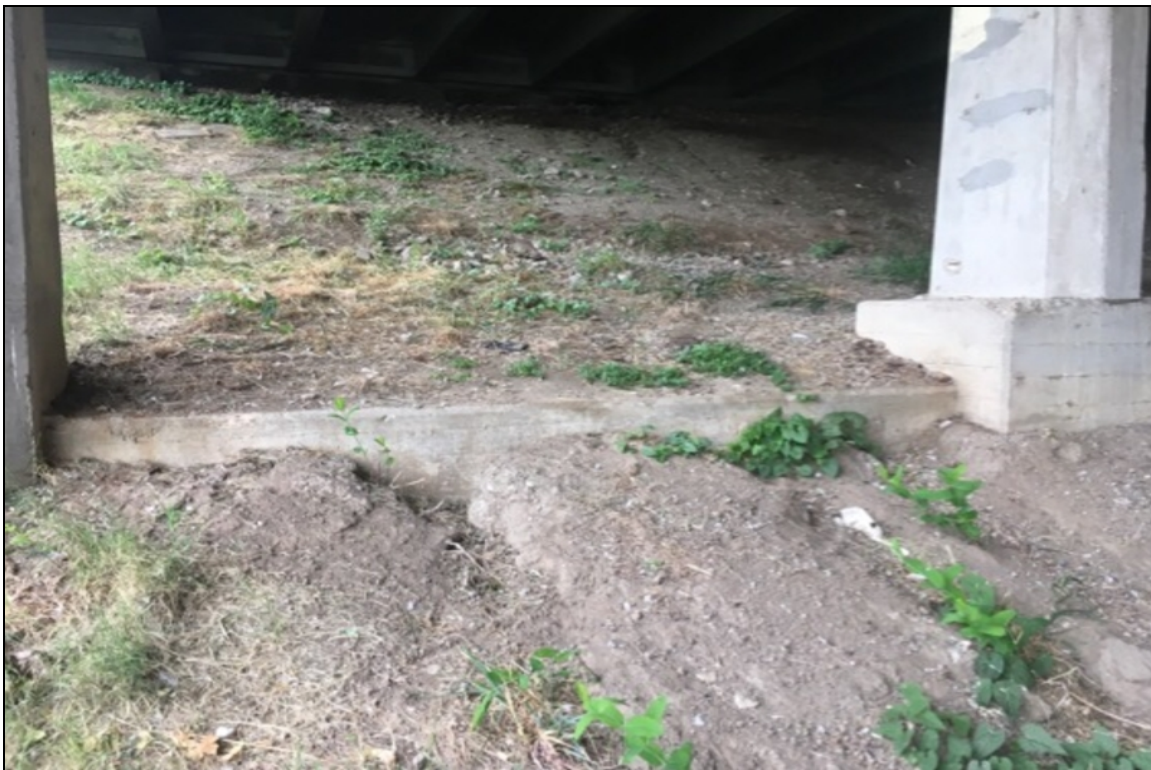
Bent 2, Footing: Spalling.
