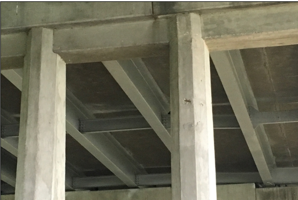
Bent 19, Column 3: Spalling with exposed reinforcing steel.
