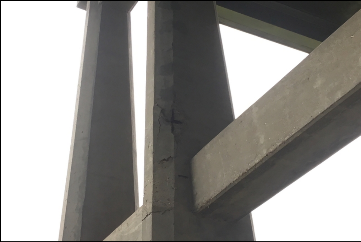
Bent 14, Column 5: Spalling with exposed reinforcing steel.
