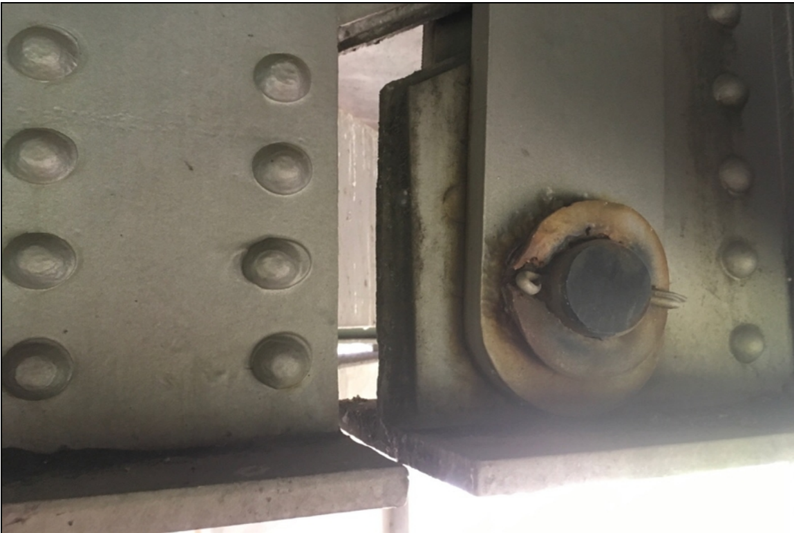
Span 10, Girder 6, Bottom Pin, Washer: Rusted through.
