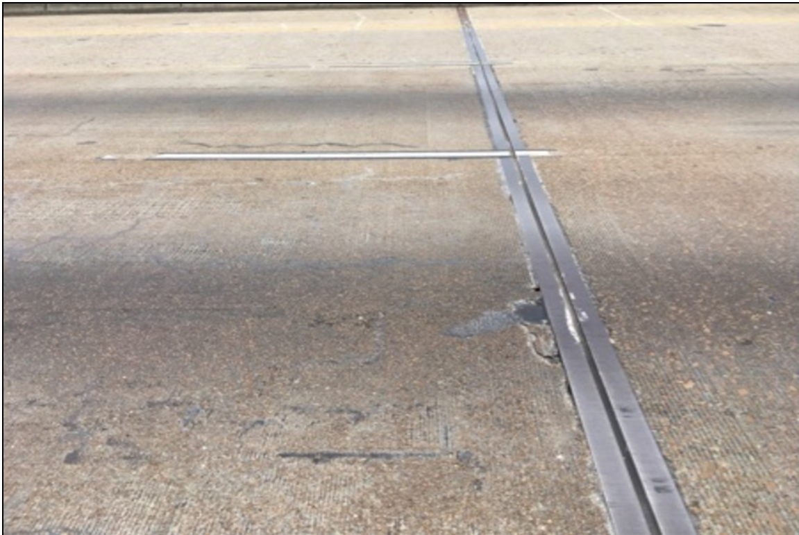
Span 1: Failing repairs.
