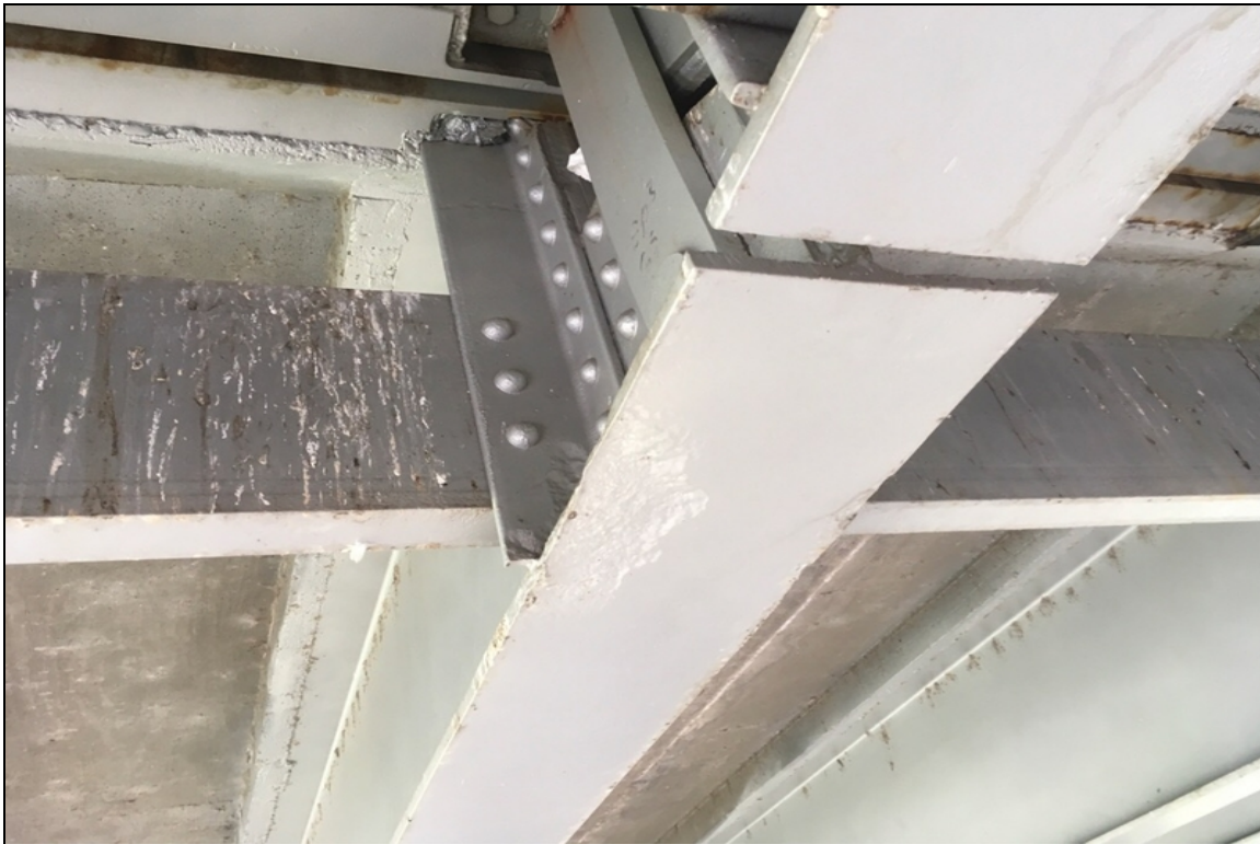
Span 3, Girder 5, Bottom Flange: Section loss.
