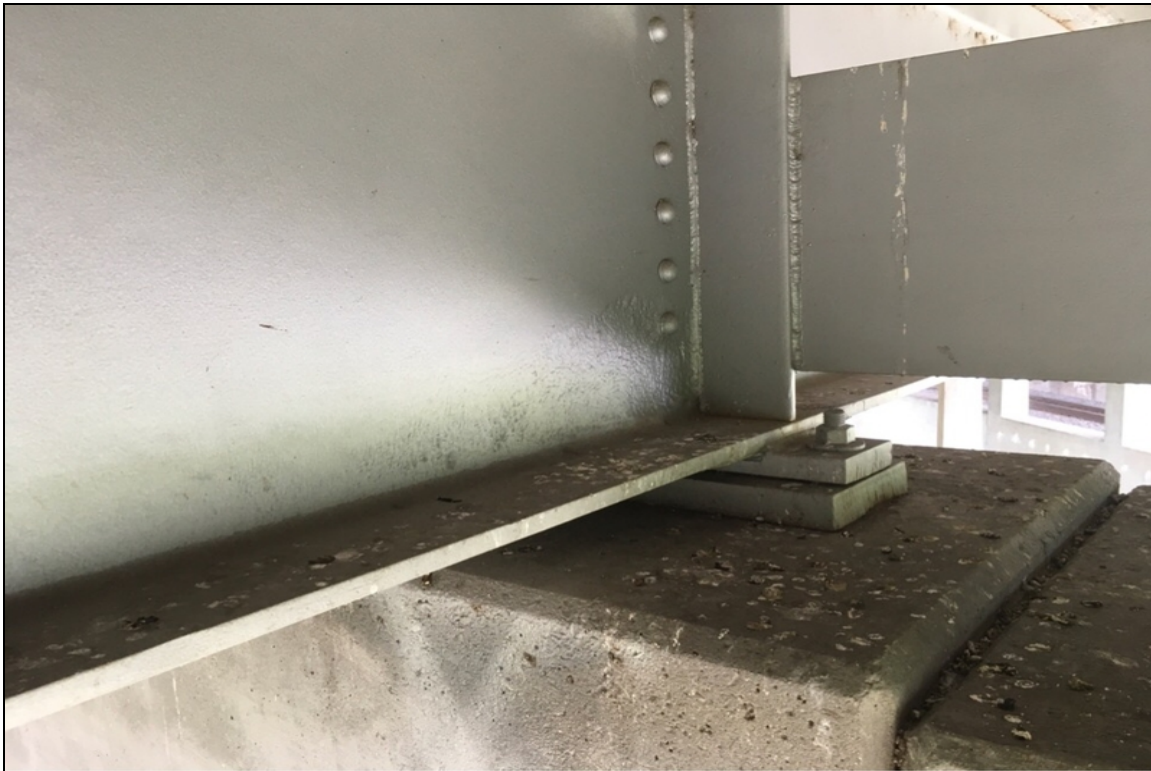
Bent 9, Girder 8, Web: Section loss.
