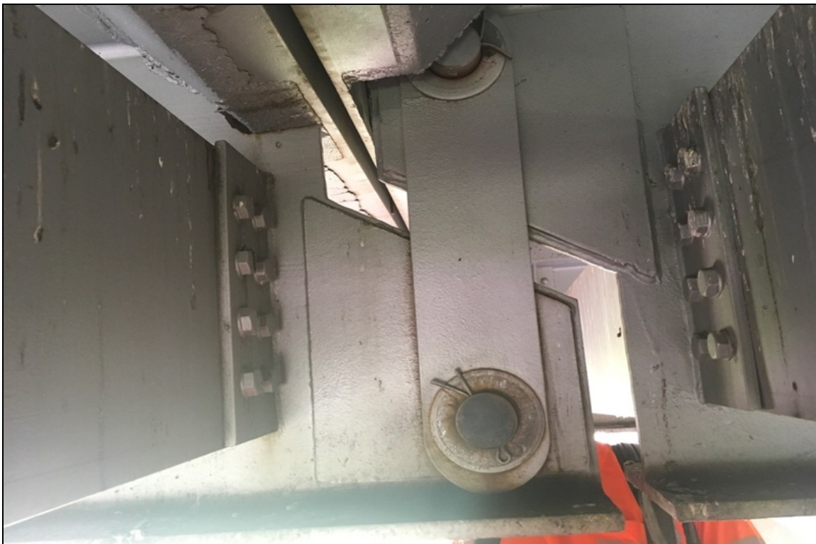
Span 21, Girder 4, Pin & Hanger: Floating.
