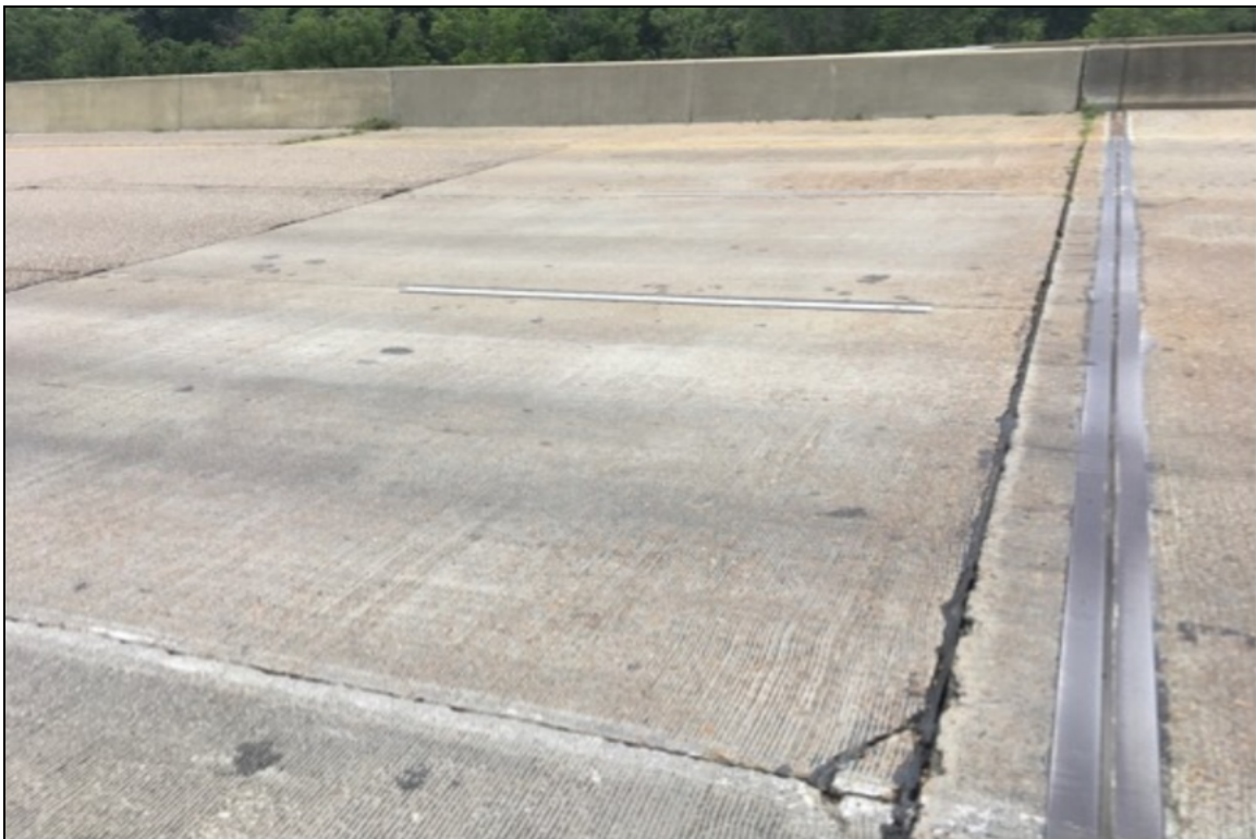
Approach 1: Spalling.
