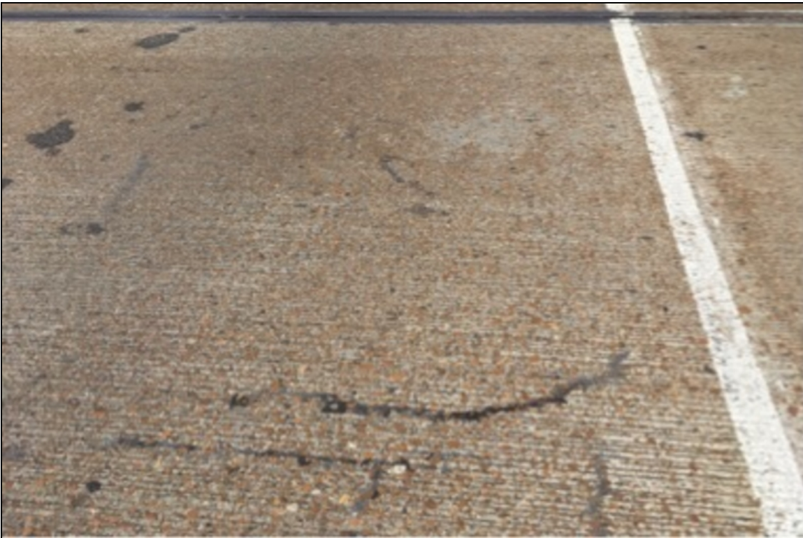
Span 6: Sealable deck cracking.
