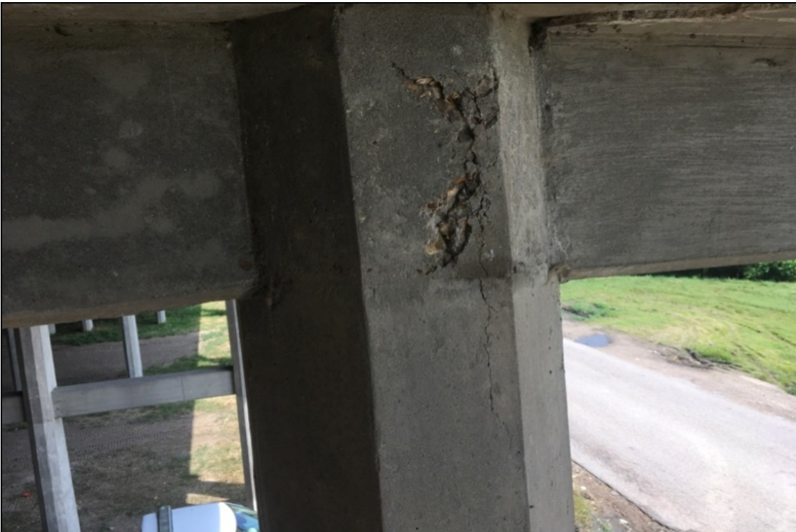
Bent 5, Column 5: Minor spalling.
