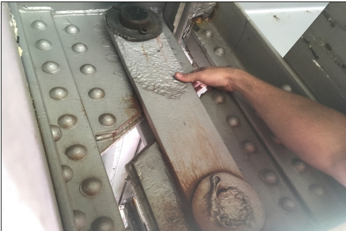
Span 9, Girder 6, Pin & Hanger: Floating.
