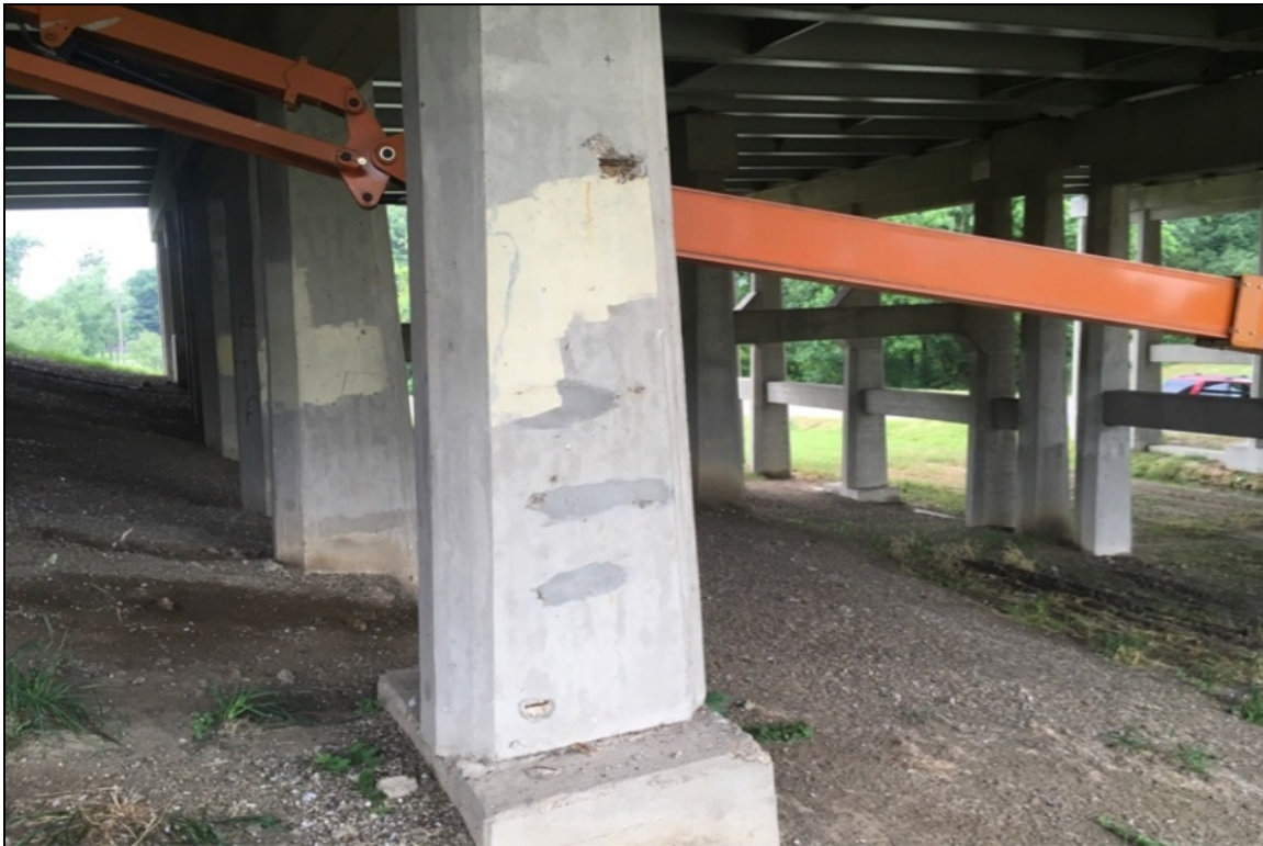
Bent 2, Column 4: Spalling with exposed reinforcing steel.
